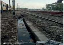
Figure 4.1: Sewage of Platform No.03/04 blocked with Ballast at Gaya (ECR).
